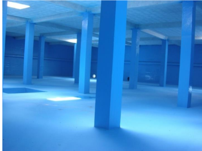
Photo: Drinking water tank waterproofed with Polyurea Rayston in Guadalajara (Spain).
