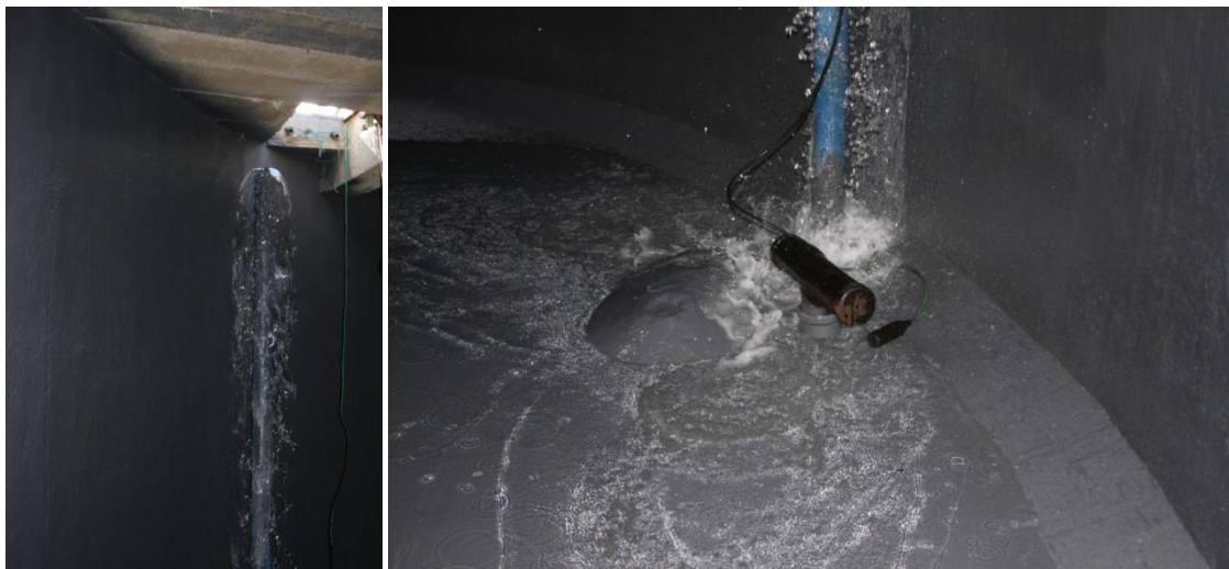
Photo: Filling a drinking water tank in Killone, Ireland after treatment with Polyurea Rayston.
