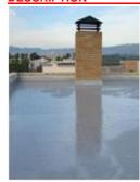
One component liquid waterproofing composition, after polymerization gives an elastomeric, cold-applied polyurethane membrane. Slightly thixotropic, low sagging product.
