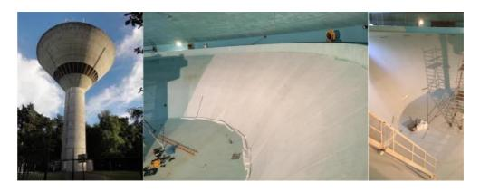
6) Drinking water tank System: Epoxy 100, Impermax Aqua 2K. Surface: 800 m<sup>2</sup>.
